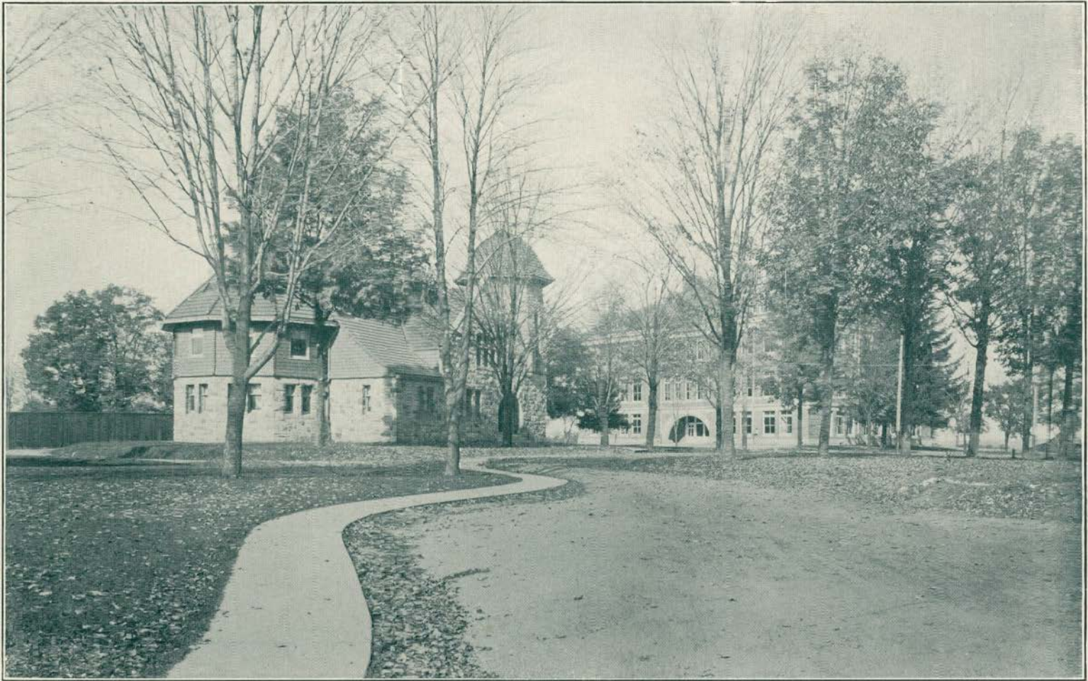
SC ENCE BUILDING AND STARKWEATHER HALL
