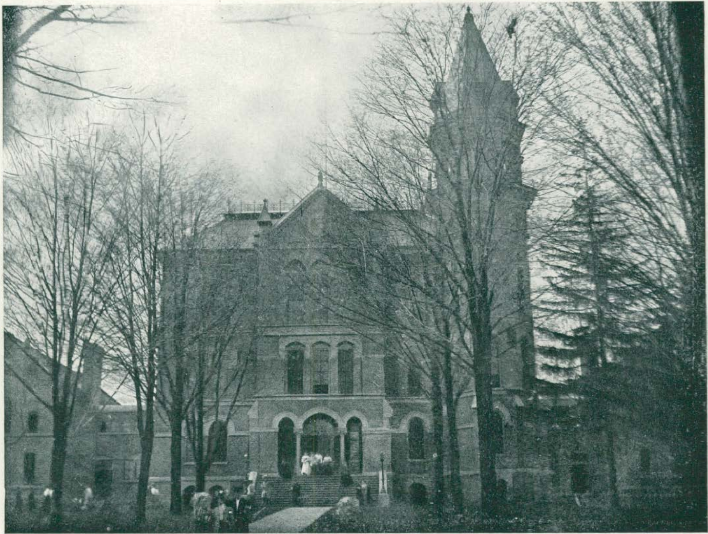
Front View Main Building
