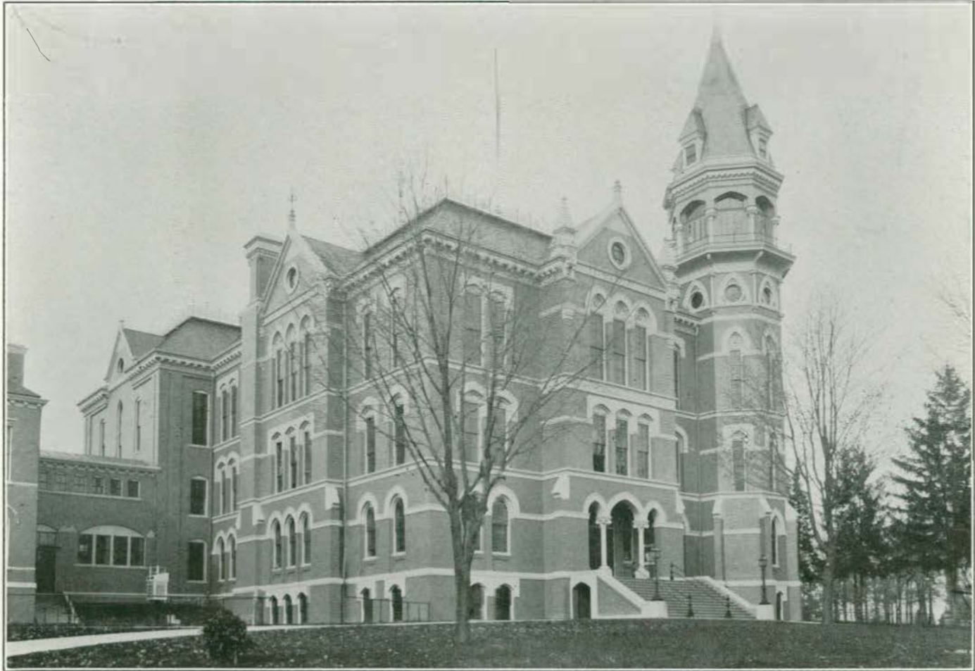
Front View of Main Building
