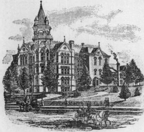
Main Building After Front Addition, 1878.
