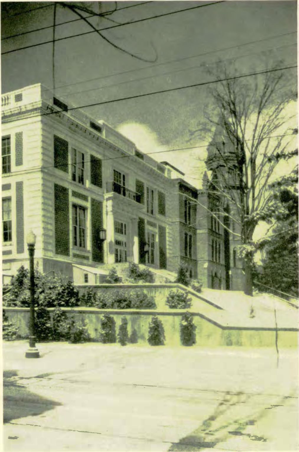
Administration Building and Normal Hall
