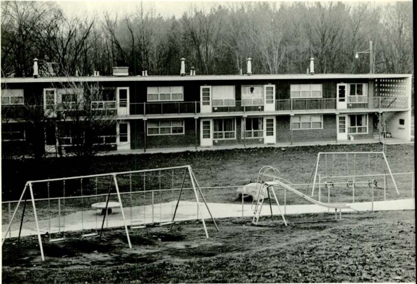
A view of Pine Grove Terrace showing also the play area provided for the children of the residents.
