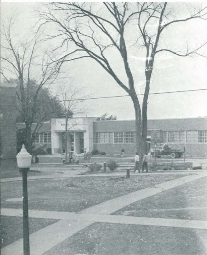
First step in renovating McKenny was the removal of trees.
