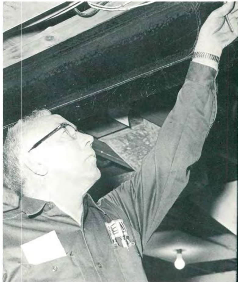
Physical Plant Worker completes electrical job.
