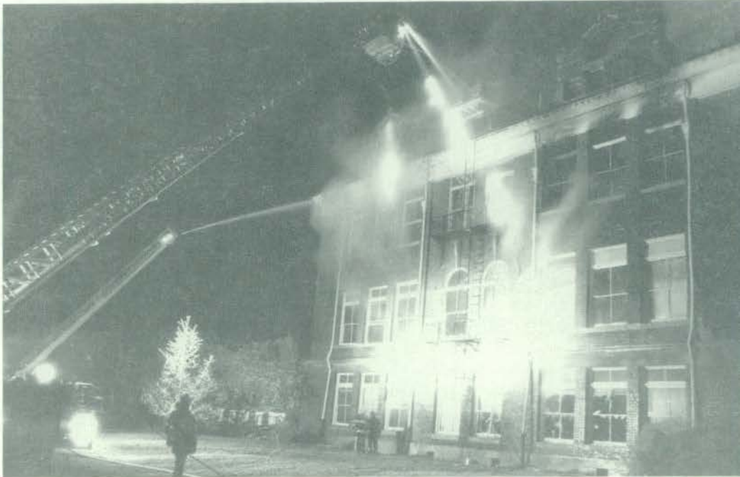
Firefighters began arriving at the scene within minutes of the initial call, but the fire had spread so rapidly that they were unable to enter the building. —Nelson
