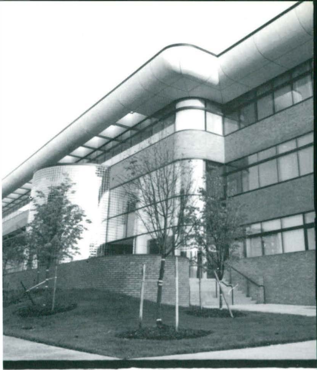
The Gary Owens College Of Business is located off campus in downtown Ypsilanti, making it a commute for all students. Finished in winter of 1991 the school took three years to build.
